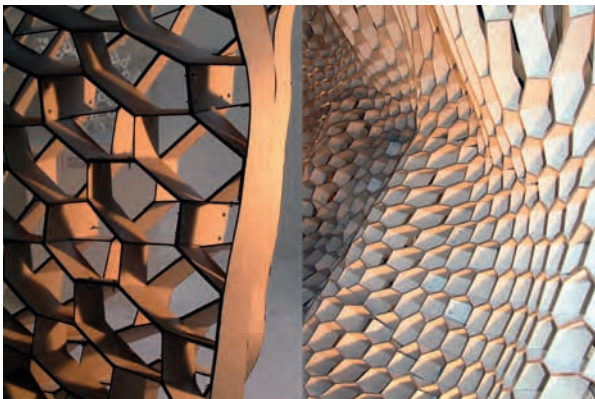
Master-project by Andrew Kudless, EmTech (Michael Hensel, Achim Menges, Michael Weinstock), Architectural Association. Generative algorithmic definition, close-up views showing planar connection tabs between honeycomb layers (left) and double-curved global surface articulation (right). Left: Photograph © Sue Barr/AA; Right: Photograph © Achim Menges.
